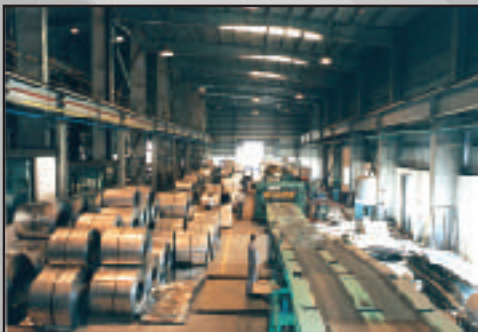
Continuous NOF Galvanizing Plant
