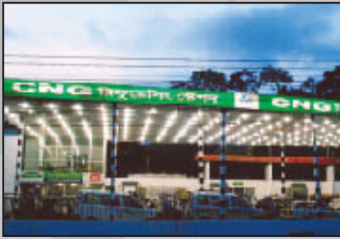
CNG Refuelling Station
