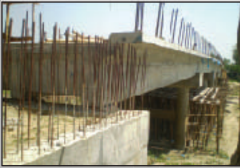
Bridge Construction Project
